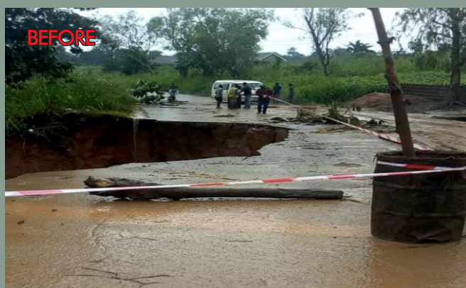
ANAMBRA STATE (Reinstatement of Massive Washout at Km 29+500 along Oba-Nnewi-Okija Road, Anambra State by Direct Labour)
