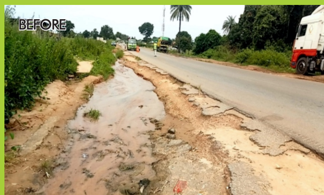
NASARAWA STATE (Direct Labour for Reinstatement of Washout and Construction of Concrete lined drains at CH.9+800 – CH.9+915 along Lafia – Akwanga Road, Nasarawa State)
