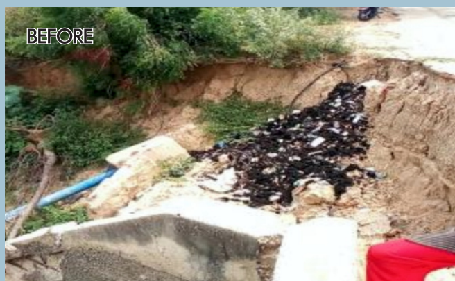
JIGAWA STATE (Emergency Repair of Washout at CH.161+025 (Malam Madori Township) along Kano S/B – Garki – Gumel – Malamadori - Hadejia Road, Jigawa State By Direct Labour)
