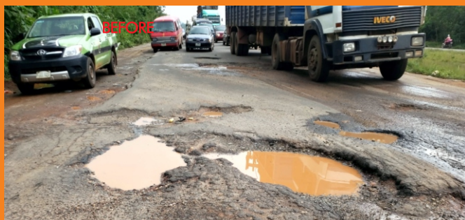
OYO STATE (Patching of Potholes/Repairs of Critically Failed Section Between KM 24+500 - KM 28+500 (Fiditi Area) along Ibadan - Oyo Dual Carriageway (Ibadan Bound), Route 20A, Oyo State)
