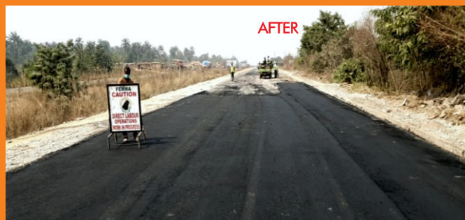
OYO STATE (Patching of Potholes/Repairs of Critically Failed Section Between KM 24+500 - KM 28+500 (Fiditi Area) along Ibadan - Oyo Dual Carriageway (Ibadan Bound), Route 20A, Oyo State)
