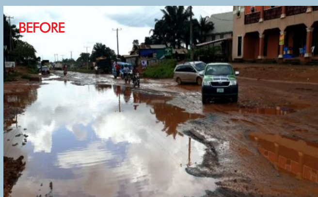
IMO STATE (Reinstatement of Failed Sections Between KM. 42+300 – KM. 55+250 along Owerri – Okigwe Road, Imo State (Umuna – Okigwe Junction Section)
