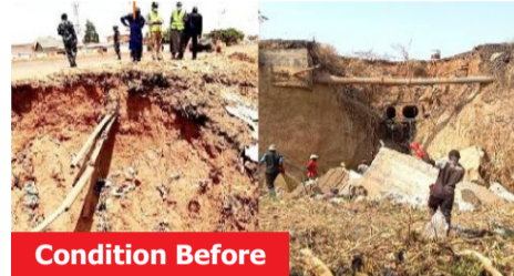
KADUNA STATE Rehabilitation of Collapsed Double Cell Pipe Culvert and Reinstatement of Embankment Washout at Ch.1+550 along Kaduna Western By-pass
