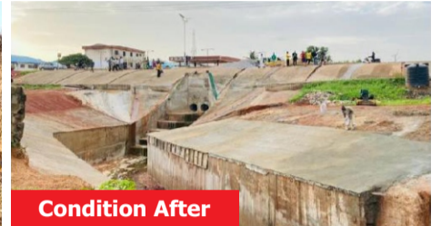
KADUNA STATE Rehabilitation of Collapsed Double Cell Pipe Culvert and Reinstatement of Embankment Washout at Ch.1+550 along Kaduna Western By-pass
